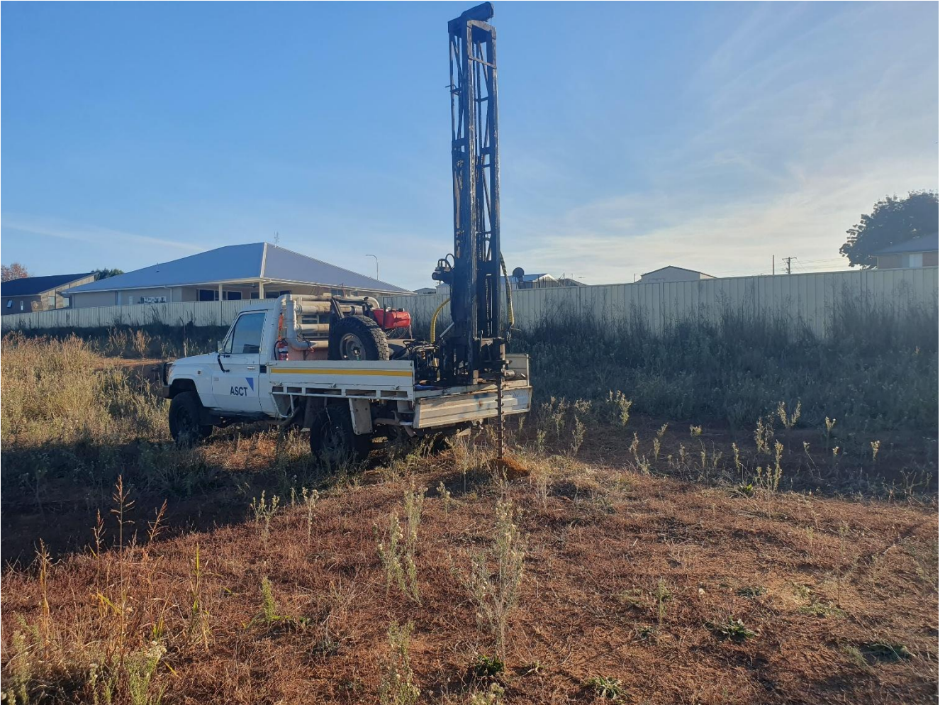
View of the site facing a south westerly direction.
